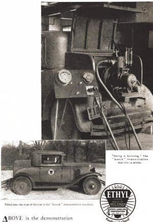
ABOVE is the demonstration machine which engineers from the Ethyl Gasoline Corporation take from place to place to prove how Ethyl "knocks out that 'knock'" and develops an engine's maximum power.
